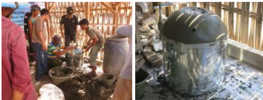
Figure 5. Construction of hong coral transplantation modules
